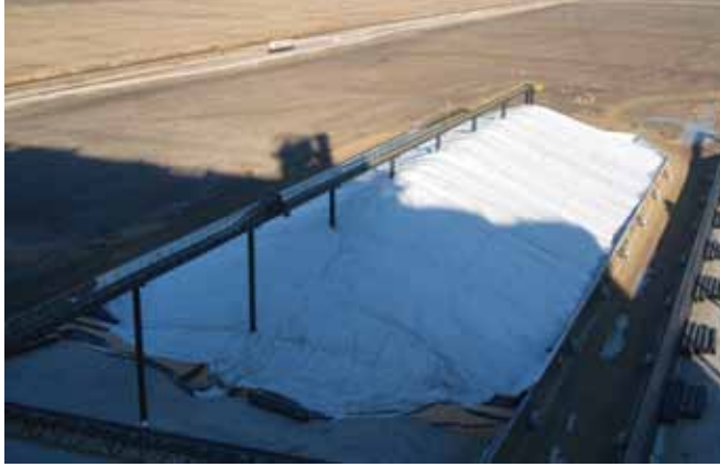
One of two 2-million-bushel temporary storage piles at the Rock Port elevator. Portion of an 8,300-foot loop track is visible in the background.
